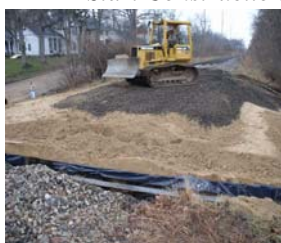
Friday Backfill & RR Base
