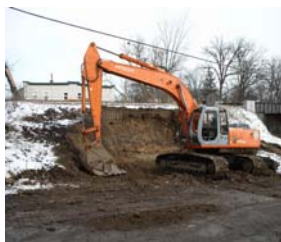
Wednesday, 11/26/03 Start Construction
