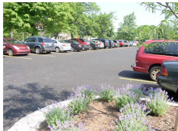
North Parking Lot Porous Pavement
