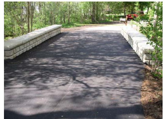
Final Residential Drive over New Culvert
