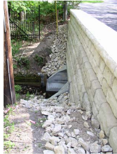
Modular Block Headwall over Box Culvert
