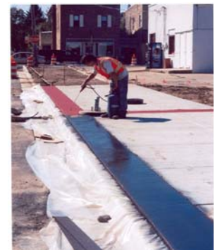
Colored Concrete with Brick Stamp Pattern
