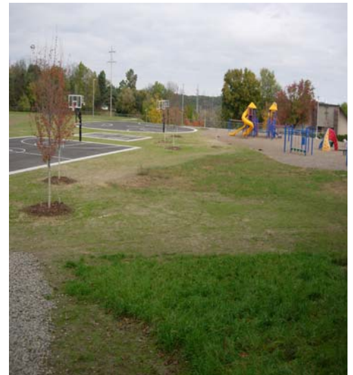
On-site stormwater storage grading
