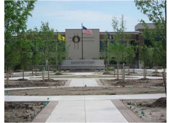
Pedestrian Plaza under construction at the new Courthouse
